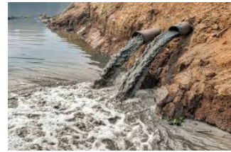
Fig. 7 Source water contaminates.
